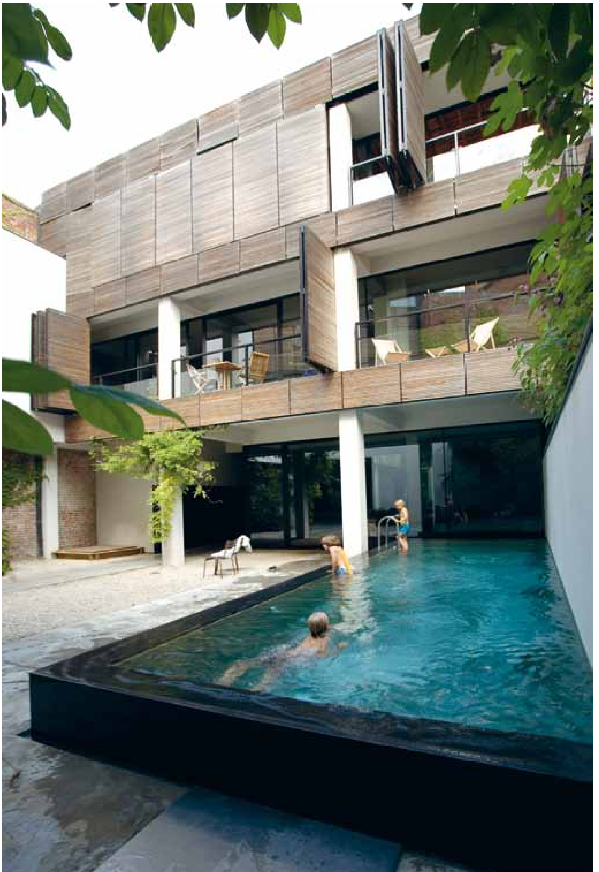
Pyrex Brussel, Architectslab
