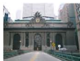
Grand Central Station (H.061)
