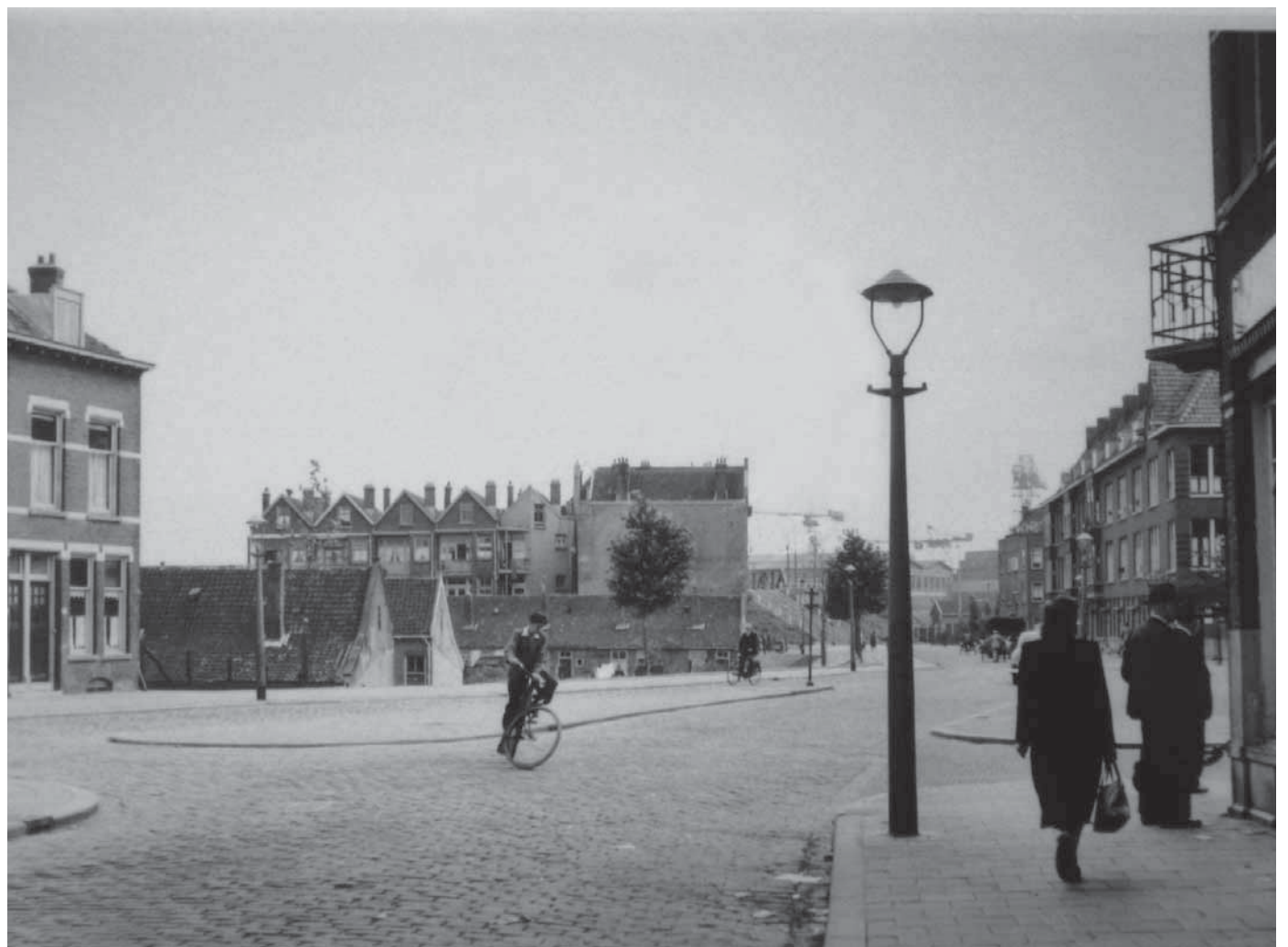
Hilleplein 30's, looking towards pedestrian bridge to the shipyards
