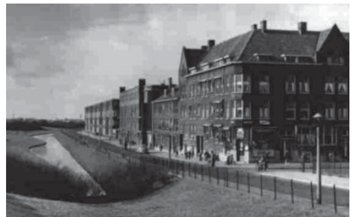
Spangen train dike, 1955
