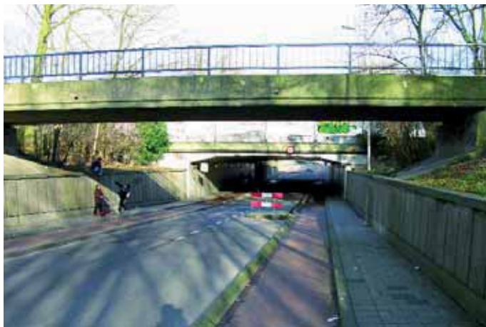
Underpass through the Sidelinge Park, current situation
